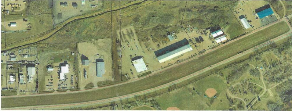
North Signage Corridor
